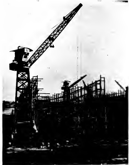
Another view of the building berths at the Alameda plant showing the start on the construction of a large steamer.
